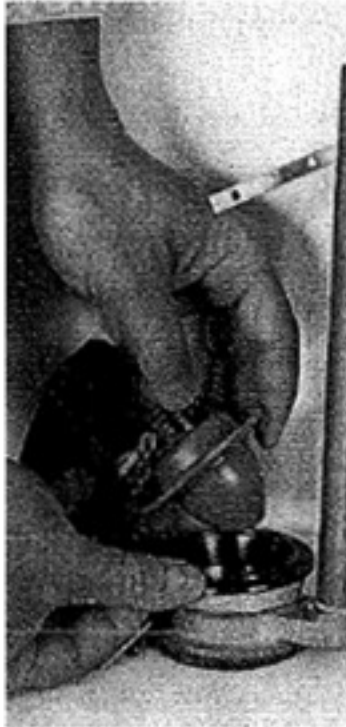
2 Press the replacement seat over the old seat.
