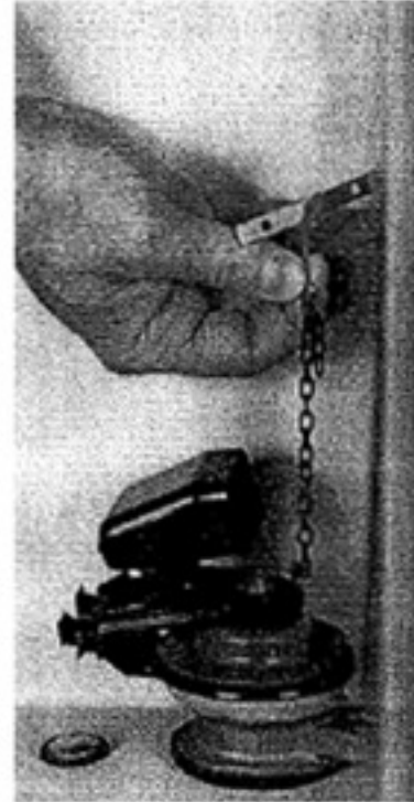
3 Connect the chain with about 1/2 inch of slack.
