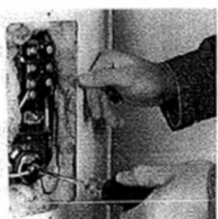
**2** Trim any charred wires, and strip the insulation back 1/2 in. Insert the wire back into its slot, and tighten the terminal screw.
