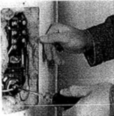
**2** Trim any charred wires, and strip the insulation back ½ in. Insert the wire back into its slot, and tighten the terminal screw.
