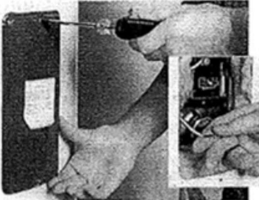
**1** With the power shut off at the electrical service panel, remove the water-heater access panel and insulation. Check for charred wires (inset).
