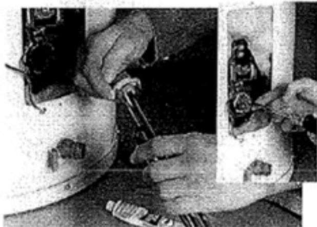
Coat the element's threads and rubber washer with pipe joint compound, and screw the element in place.
