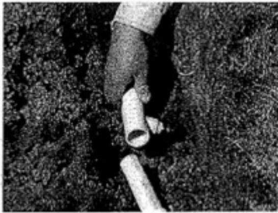
**3** To drain a supply line low point, install a T-fitting with a threaded branch. Screw a brass drain into the branch.
