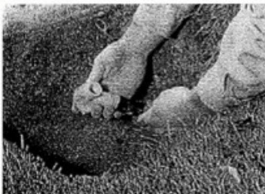
**6** When water will be trapped at the end of the line, use a self-draining ell to connect the sprinkler head.
