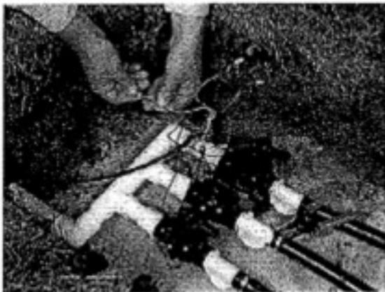
**2** With the first three zone valves ganged and piped, connect the low voltage wires to the valves with twist connectors.
