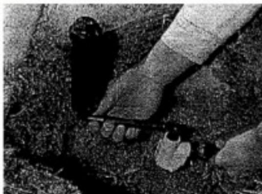
**7** Swing pipe allows you to move the head where you need it so that you can make last-minute adjustments. It doesn't need crimp rings.
