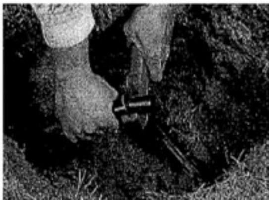
**4** Use a scissor-style pipe cutter to slice through polyethylene pipe. Push the pipe into the fittings until they bottom out on the barbs.
